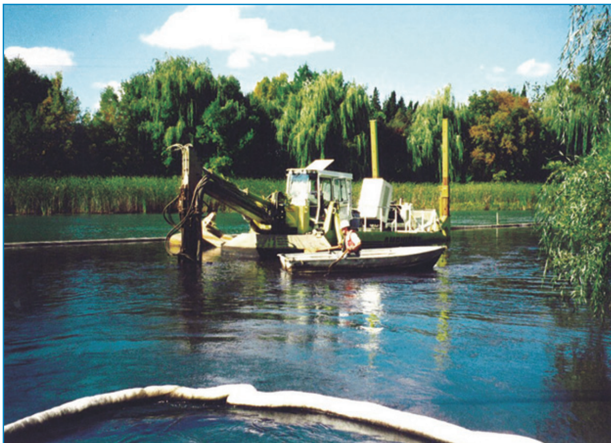
Figure 7: Dredging deposits of mill-scale at the Welland River reef site in 1995
