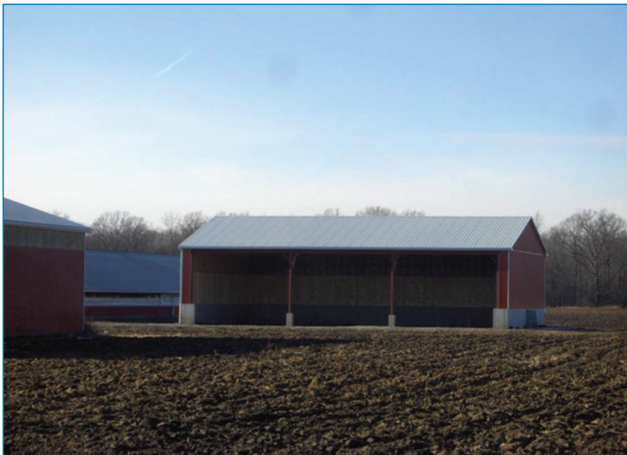
Figure 6: A new manure storage facility in the Niagara River AOC
