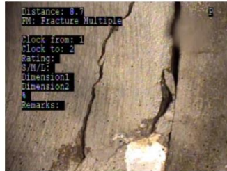
Davy St., Storm - Fractures Multiple
