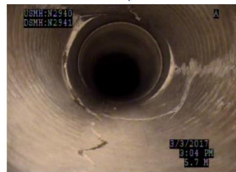
Platoff St., Storm - Broken
