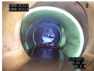
Platoff St., Storm - Joint Offset Large
