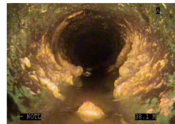
King St., Sanitary - Settled Gravel
