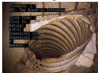
King St., Storm - Defective Tap
