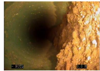
King St., Sanitary - Grease Deposits
