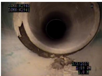
Platoff St., Storm - Joint Offset
