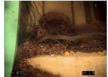
King St., Sanitary - Heavy Roots
