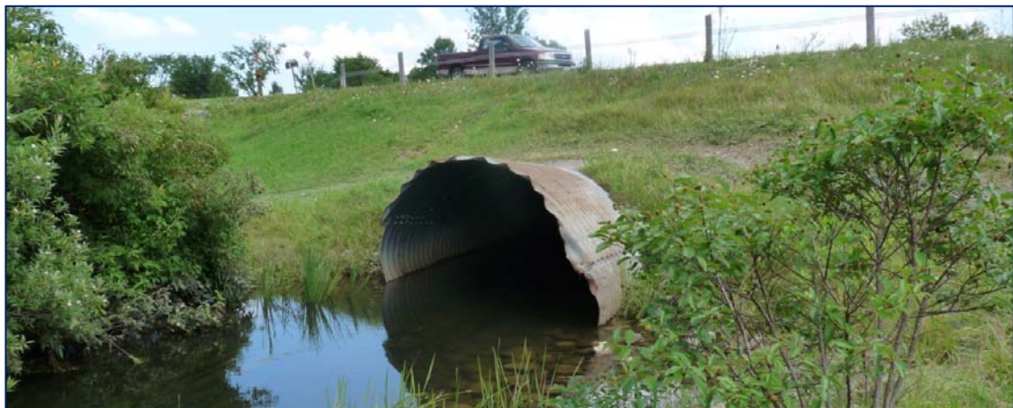
Lyons Creek East - Zone 3 - Culvert at Highway 140
