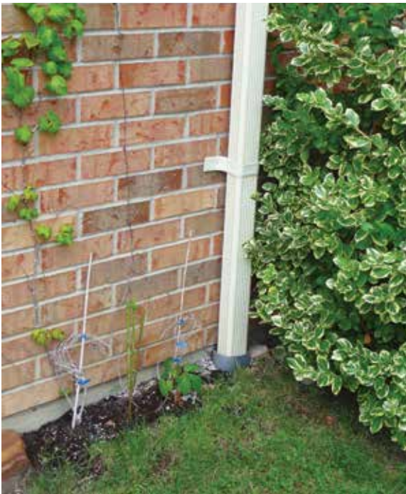
Downspout Connected to Storm System
