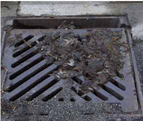
Typical Storm Drain
